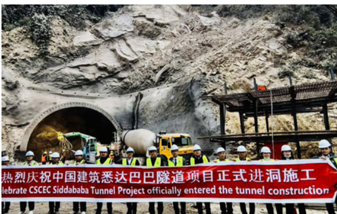
Fig. Portal of Siddhababa Tunnel (Source: My Republica, post on June 18, 2024)
